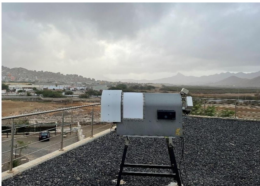
Figure 28: The RPG microwave radiometer installed on the rooftop of the OSCM, Cape Verde.
